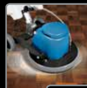
Wooden floor sanding
