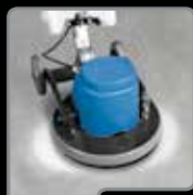
Smoothing and restoration of concrete screed
